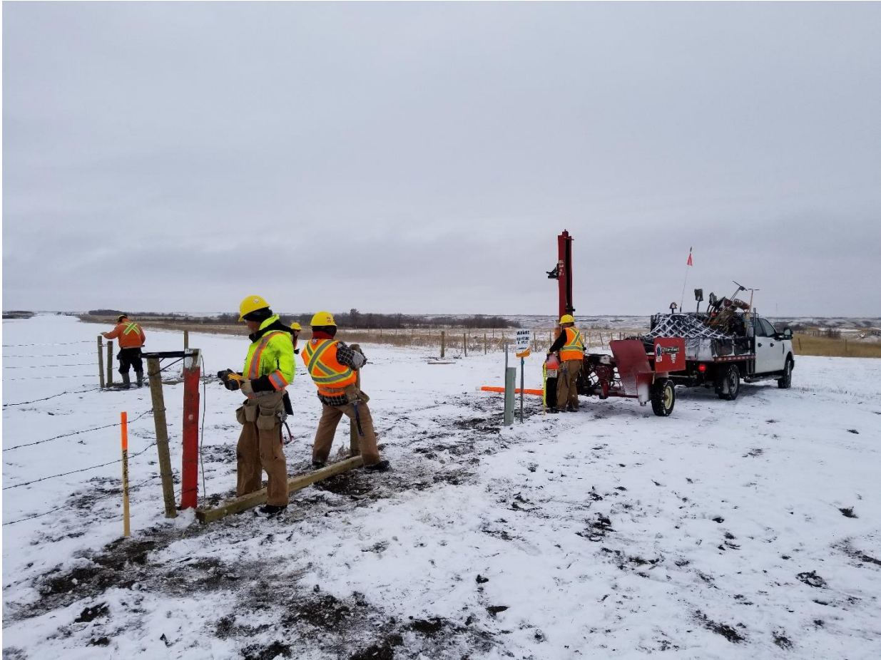
Utility installing new fence and new gate.
