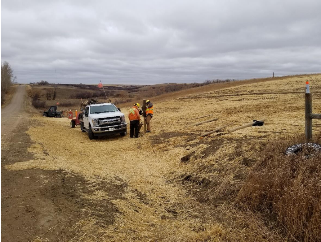
Utility crew fencing off the road at High Hill Creek.
